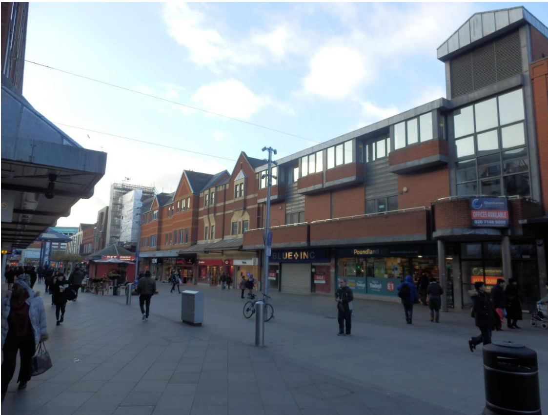
No.46 and other adjacent properties to the west
